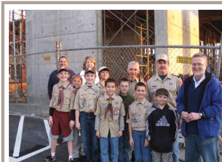
Cub Scouts Pack 105 are earning their engineering activity badge by learning how the new City Hall is being built.
