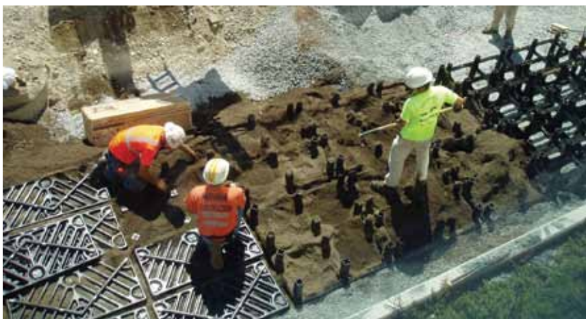
This Silva cell system of modular blocks holds lightly compacted healthy soils in place, promoting root and tree growth while bearing loads for above ground streetscapes. The underground system provides stormwater management allowing filtration to remove pollutants while retaining runoff to mitigate flooding and erosion.
