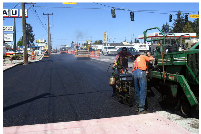
First layer of paving on west side of Aurora from N. 155 th to 165 th Streets
