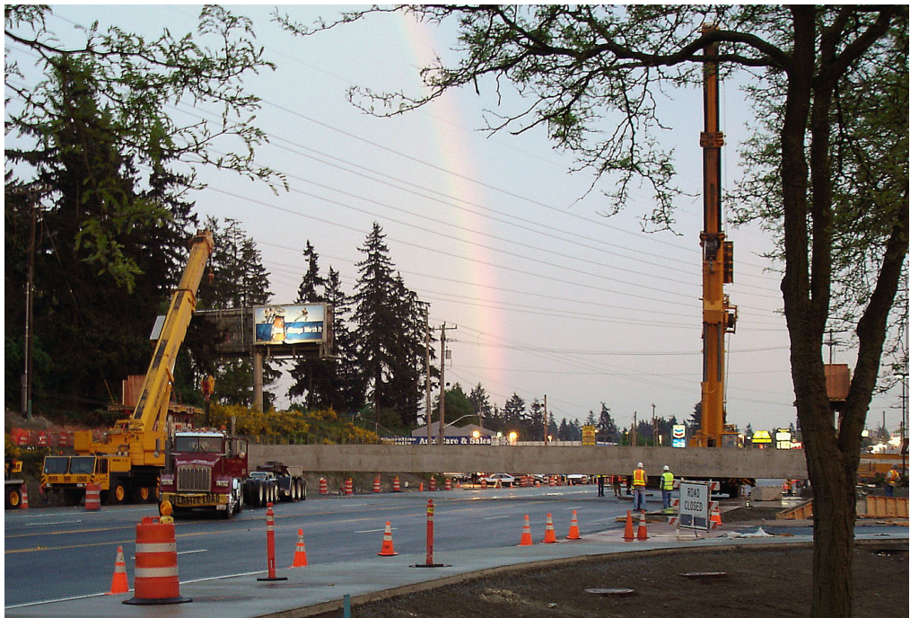
Crews set the two girders for the Aurora Interurban Trail Bridge the evening of May 19. Shoreline residents and business owners gathered to watch the historic event in the parking lot of Aurora Square Shopping Center. The girders for the N. 155th Street bridge will be set sometime this summer.
