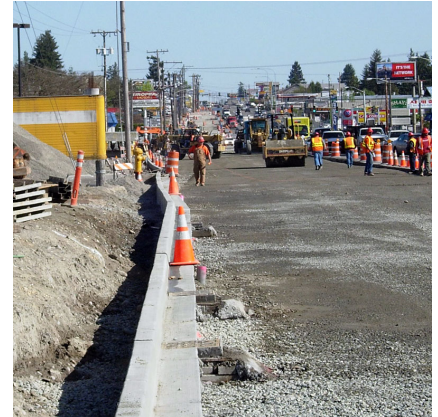
Curb/gutter on west side of Aurora between N. 145 th to 165 th Streets and shifting traffic to the west side of Aurora
