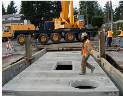
Storm water quality treatment system including filtering chambers
