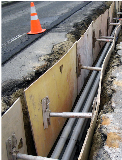
Utility vaults and conduits installed on west side of Aurora
