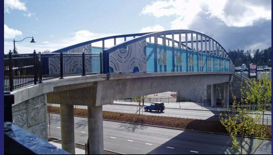
Interurban Trail bridge over Aurora
