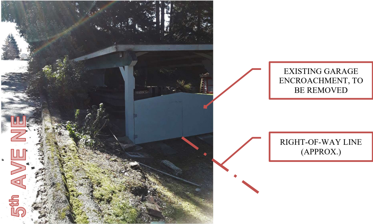
Figure 1: Existing Garage Encroachment at 361 NE Serpentine Place
