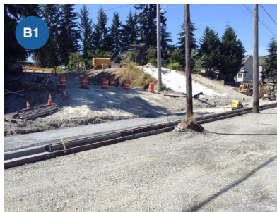
B1/B2. Curb and gutter formwork and concrete pour
