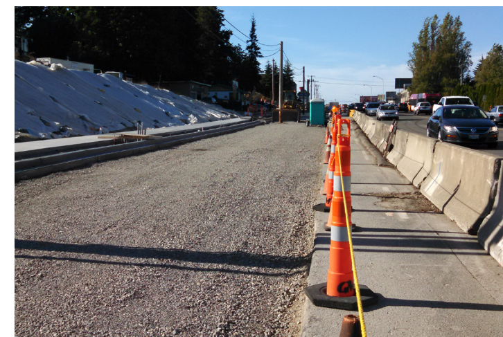
Roadbed with rock base
