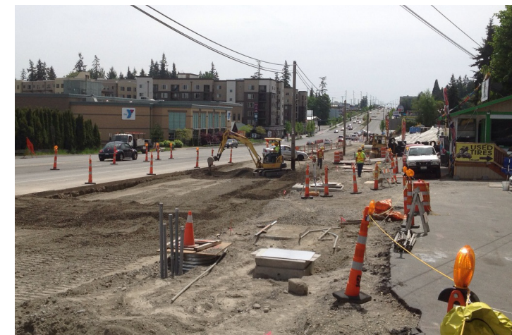
Roadway excavation and grading
