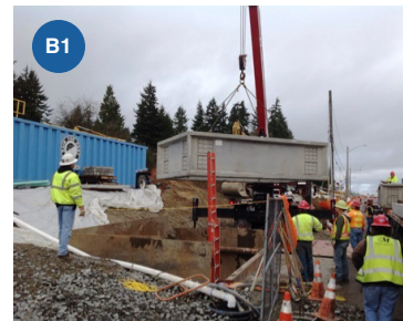
B1/B2/B3. SCL vault, cover, and lid installation
