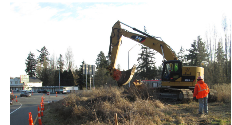
Starting to clear vegetation near N 195th Street
