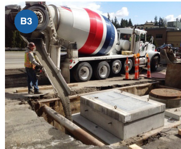
B1/B2/B3. SCL vault, cover, and lid installation
