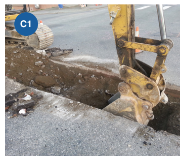
C1. Starting to excavate the trench
