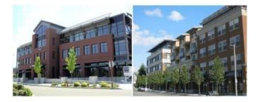
Facade Widths Using a Combination of Facade Modulation, Articulation, and Window Design
