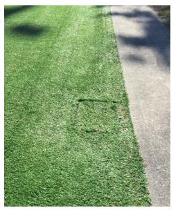
Construction traffic over quick coupling valve locations has depressed and damaged some of the boxes around the perimeter of the field. Potential damage to the valve, riser assembly, and mainline could exist.
