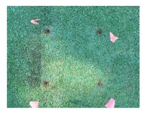
The stakes utilized at the anchor plates have created perforations, holes, and tears in the synthetic turf backing. These areas will create uneven footing and traction and will need to be repaired. They are also unsightly with some residual dirt and rust.
