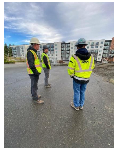
Site Visit By Owner
