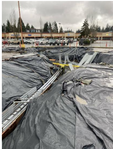
Swich Area Working
