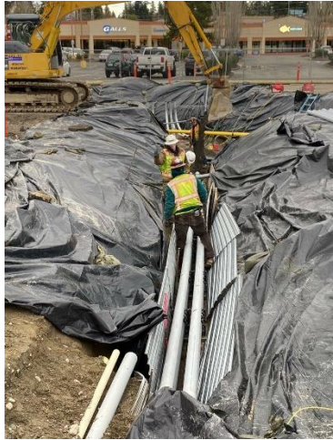
Form Power Conduits Down C. St
