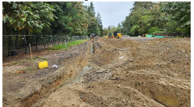
Stormwater Drain being installed at Shoreview
