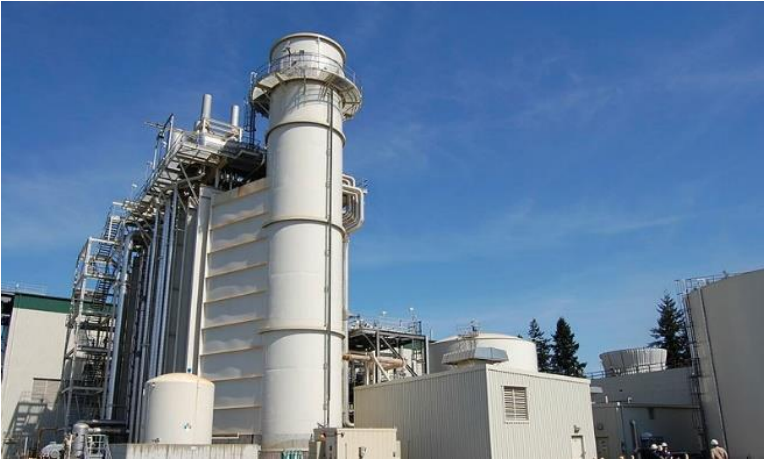
PSE's Frederickson generating station is an example of a dispatchable energy resource
