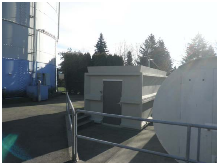
Figure 10 – Dayton Pump Station Exterior
