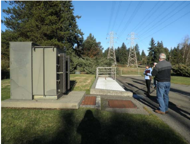
Figure 7 – North City Pump Station Exterior
