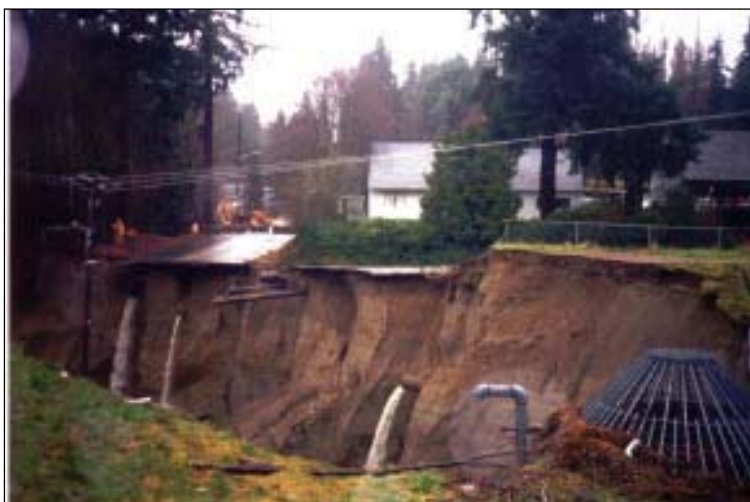
Holiday Blast Storm Sinkhole - Shoreline
