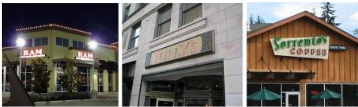
Individual backlit letters (left image), opaque signs where only the light shines through the letters (center image), and neon signs (right image).
