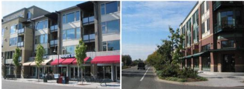
Storefront and boulevard buildings
