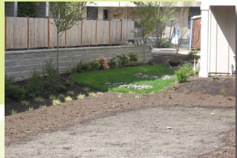
Natural landscaping at Shoreline Townhomes on Echo Lake. Grass bioswale connects driveway to new raingarden.
