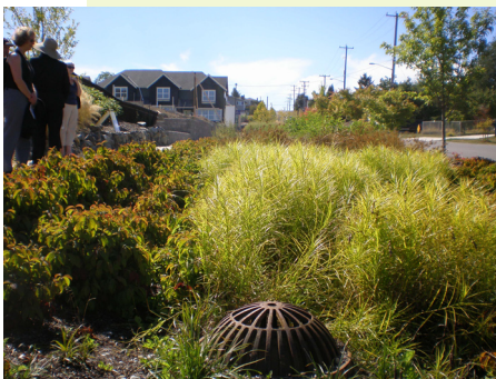
A vegetated swale at High Point in West Seattle.
