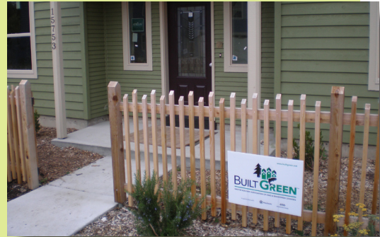
A 5-Star “Built Green” residence in Shoreline.
