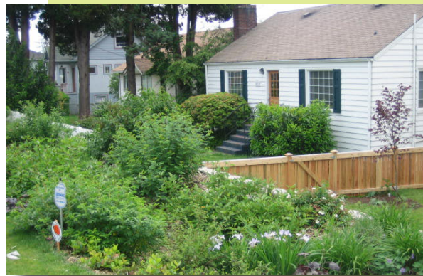
Right-of-way landscaping merges with private landscaping in Seattle.
