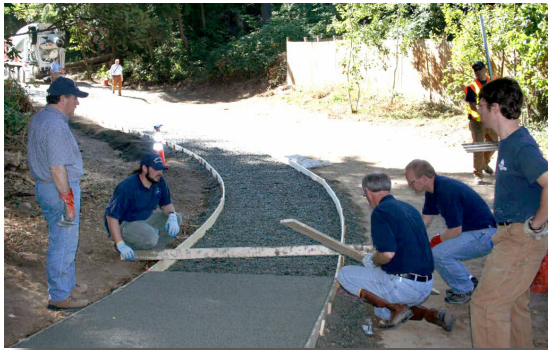
Porous concrete trail at Fremont Place in Shoreline.
