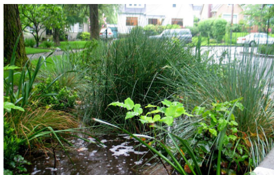
Drainage swale in Portland, OR.
