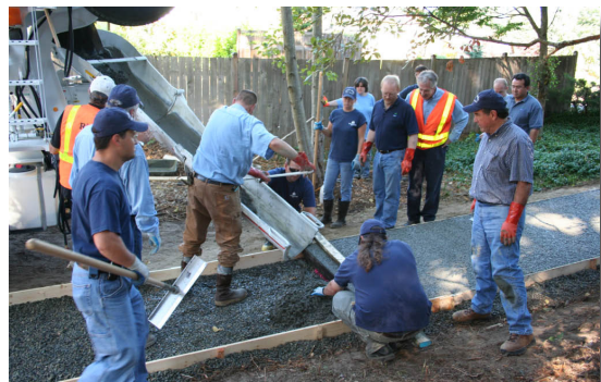
Constructing a porous concrete trail along Fremont Place.
