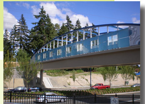
The Interurban Trail crossing Aurora Avenue.
