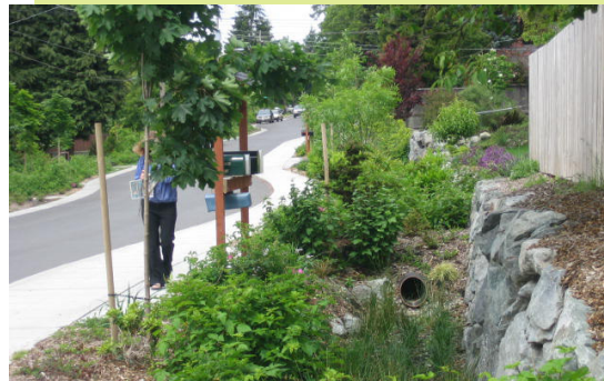
A vegetated swale along a street in Seattle is an example of Green Infrastructure.
