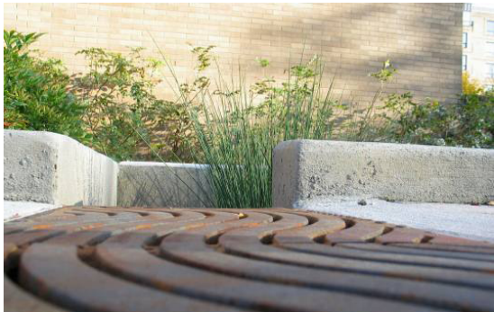
Decorative grate connected to a vegetated swale.
