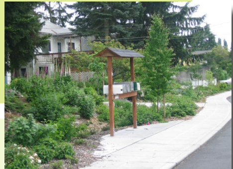
Natural landscaping and drainage edge along SEA-Street in Seattle.
