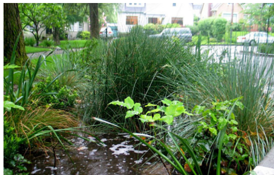
Drainage swale in Portland, OR.
