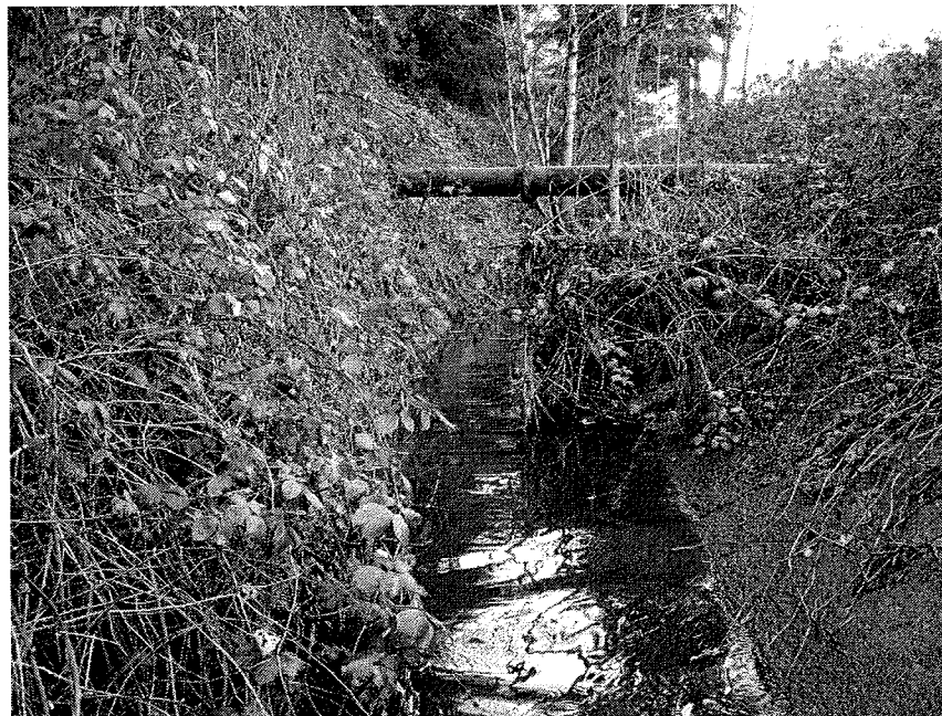
Photo 2, facing northward, upstream, showing a pipeline crossing near the north property boundary.
