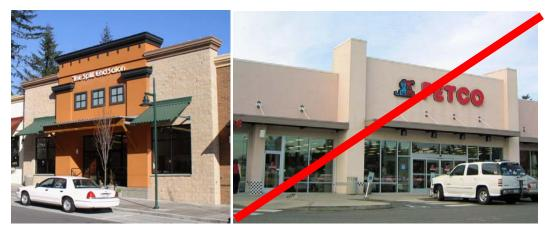
Figure 20.92.200(D). Acceptable (left) and unacceptable (right) use of synthetic stucco. The left image employs concrete near the ground level and a variety of other surface materials on the façade. The right image uses synthetic stucco for more than 50 percent of the façade and some surfaces extend to the ground level.
