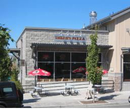
Figure 20.92.200(C). Acceptable use of concrete block on facades. The left image uses smooth gray blocks on the vertical columns and beige split-faced blocks above the awnings. The storefront in the right image uses gray split face (but less than 50 percent of the façade) and some lighter, square, smooth-faced blocks below the storefront windows.
