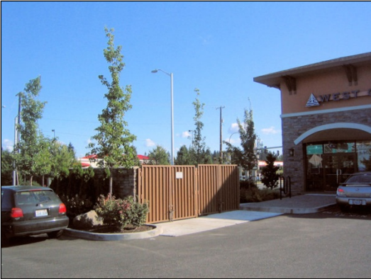
Trash/recycling closure with consistent use of materials and landscape screening.
