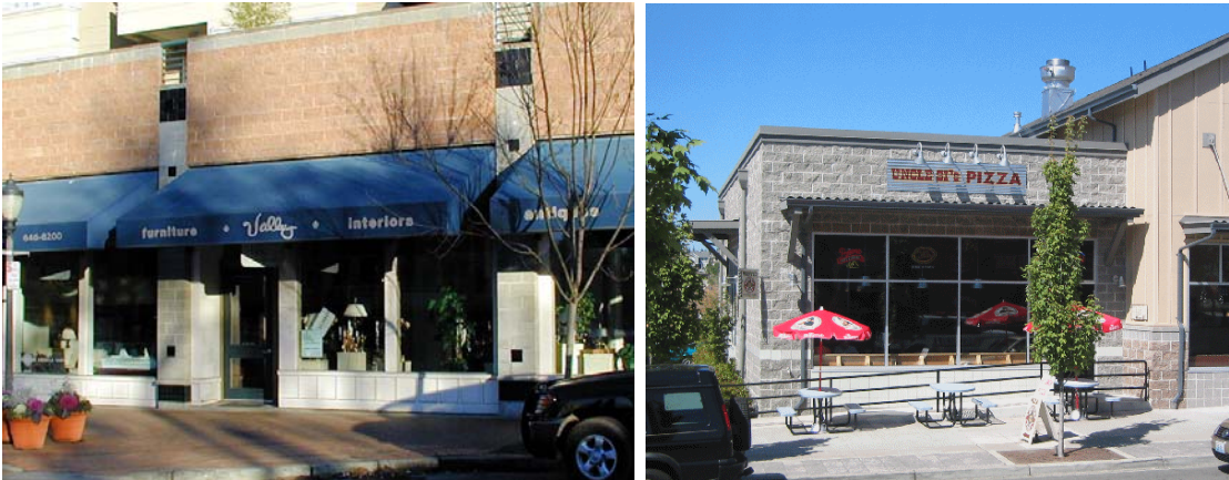
The left image uses smooth gray blocks on the vertical columns and beige split-faced blocks above the awnings. The storefront in the right image uses gray split face and some lighter, square, smooth-faced blocks below the storefront windows.
