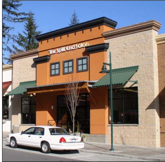
Concrete near the ground level and a variety of other surface materials on the façade.
