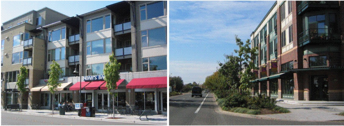
Storefront and Boulevard buildings
