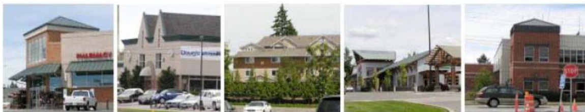
Fig. 13 Town Center roof shapes of various pitches, materials, colors
