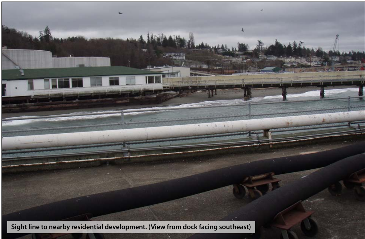
Existing floodlights at rail siding
