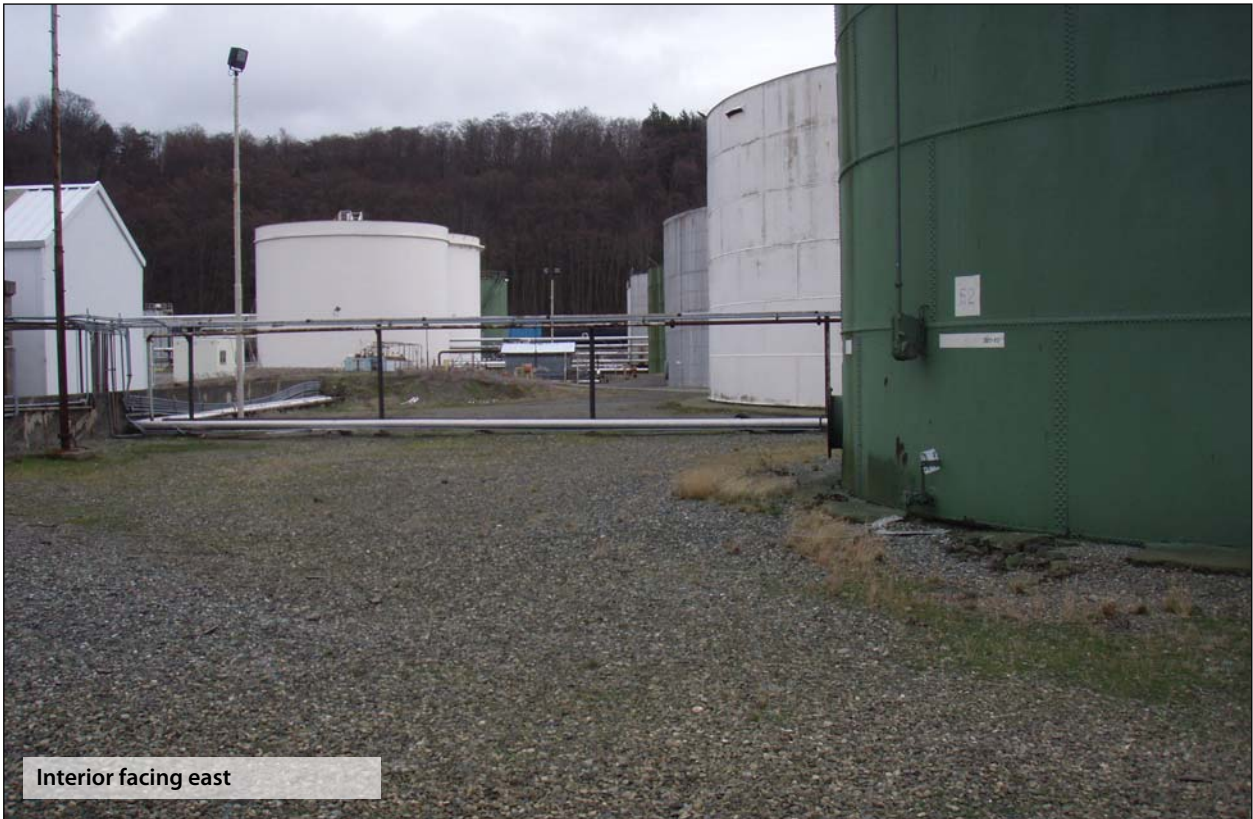
North end facing southwest
