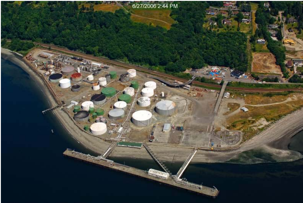
Photo A-1 View of the Paramount Washington property at Point Wells (Ecology, 2006)
