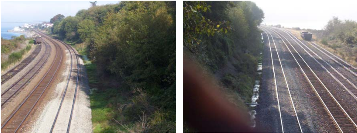
Photo C-1 Potential drainage wetlands along the BNSF railroad within Segment C
