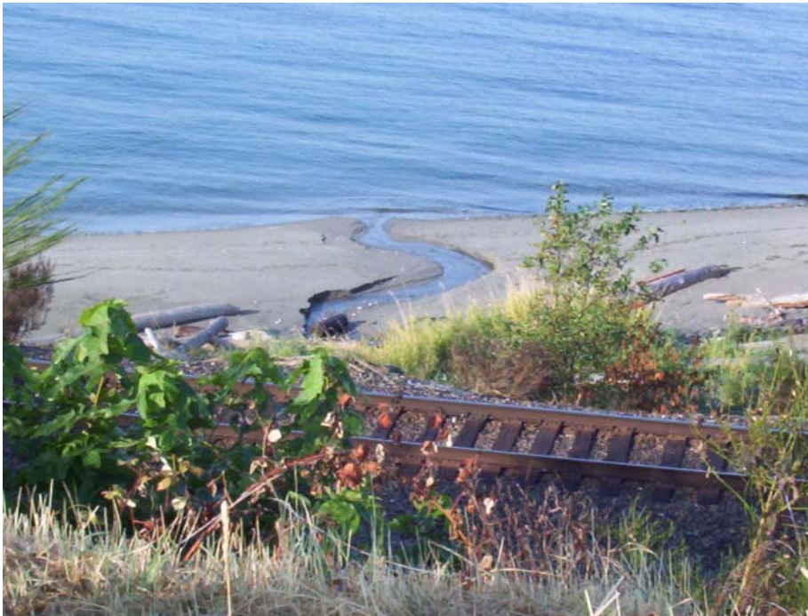
Photo B-6 Barnacle Creek outlet to Puget Sound, at southern end of Segment B
