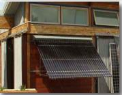
Examples of residential applications of energy efficient mechanisms and appliances, including the solar hot water collector on Shoreline Community College's Zero Energy House.
