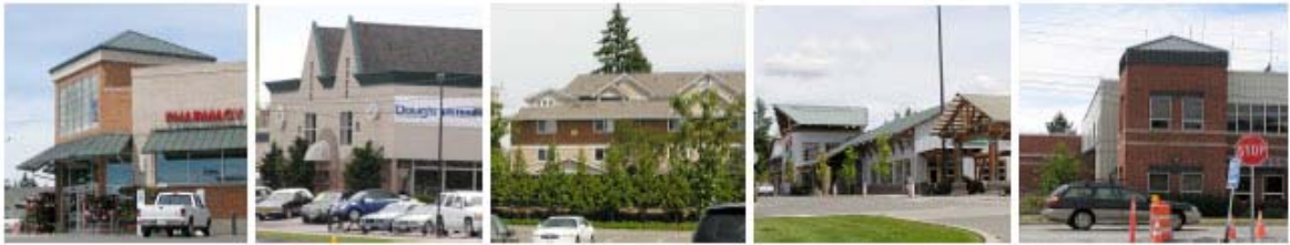
Fig. 3 Town Center roof shapes of various pitches, materials, colors
