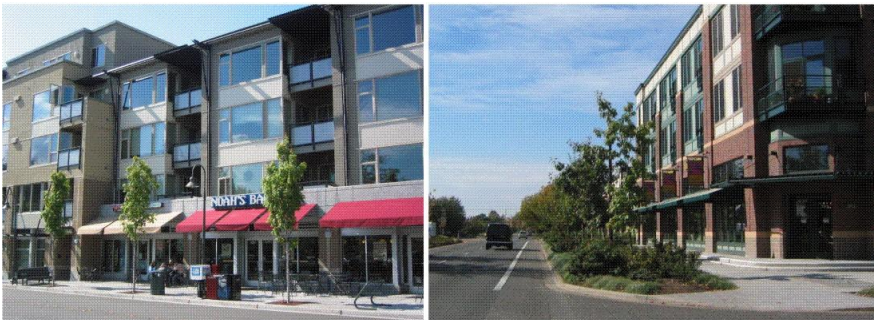
Storefront and Boulevard buildings
