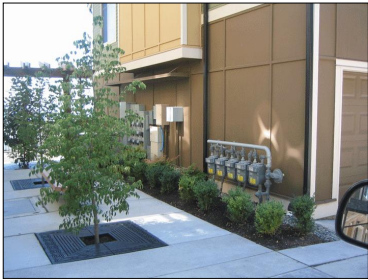
Utilities consolidated and separated by landscaping elements.
