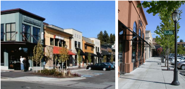
Internal walkways adjacent to storefronts should be designed to look and function like public sidewalks, including walkway widths and amenity areas.
