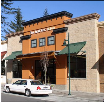
Concrete near the ground level and a variety of other surface materials on the façade.
