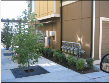
Utilities consolidated and separated by landscaping elements.
