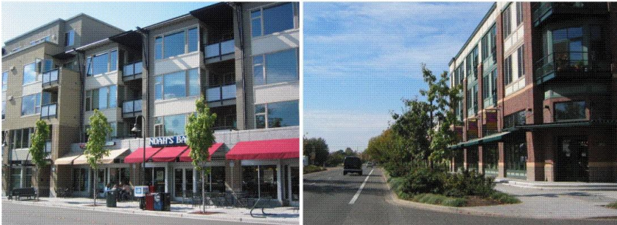
Storefront and Boulevard buildings
