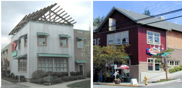
Masonry or concrete near the ground and proper trimming around windows and corners.
