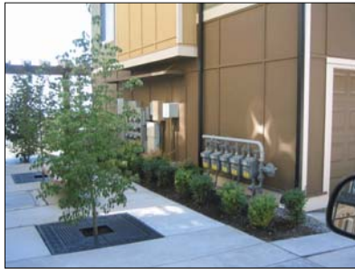
Utilities consolidated and separated by landscaping elements.
