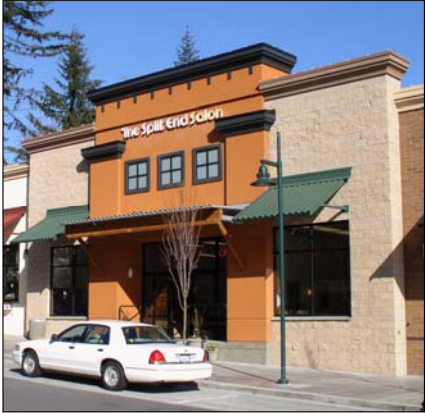
Concrete near the ground level and a variety of other surface materials on the façade.
