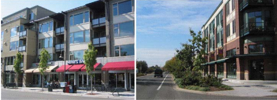
Storefront and Boulevard buildings
