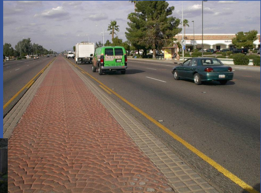
Paver Median Route 87, Chandler, AZ (Cahill Associates)
