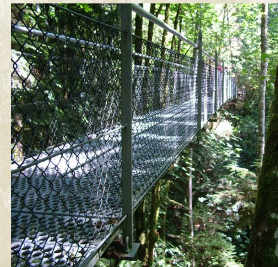
Chain link fabric and cable rail
