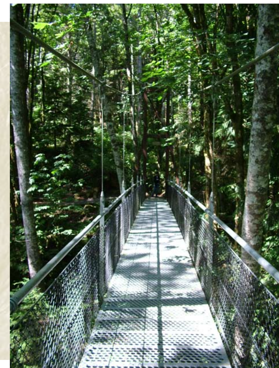
Chain link fabric and cable rail
