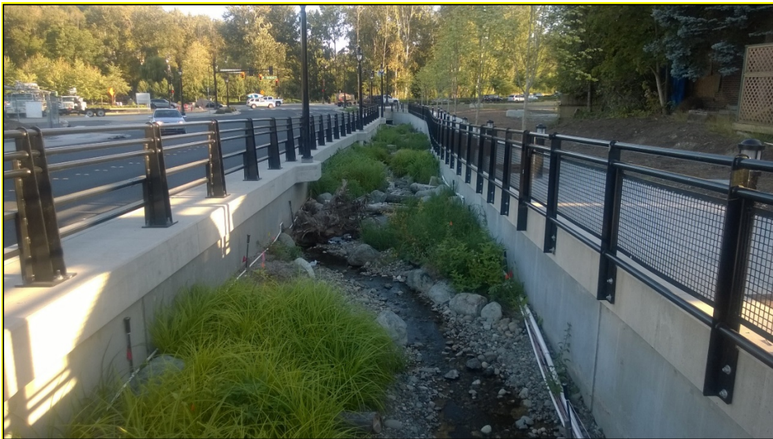
Photo 1. Example of 3-Sided Open Channel with Concrete Walls
