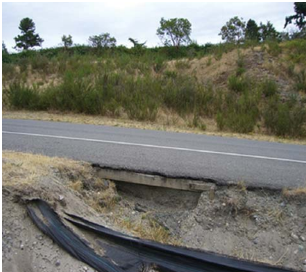
Erosion along edge of road
