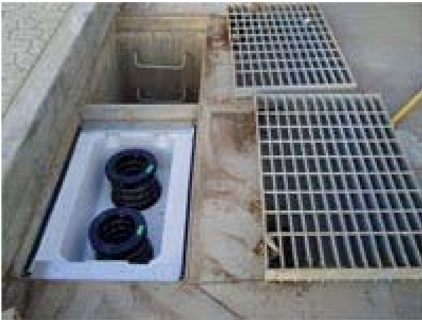
Figure 9: Stormfilter in Pre-cast Vault (Image from Contech)
