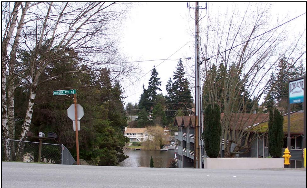
Viewpoint 6: View East from Project. Facing east from Aurora Avenue N along N 195th Street towards Echo Lake within Landscape Unit 2.
