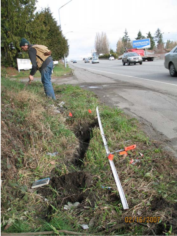
Photo 10. Ditch 1 Facing North
