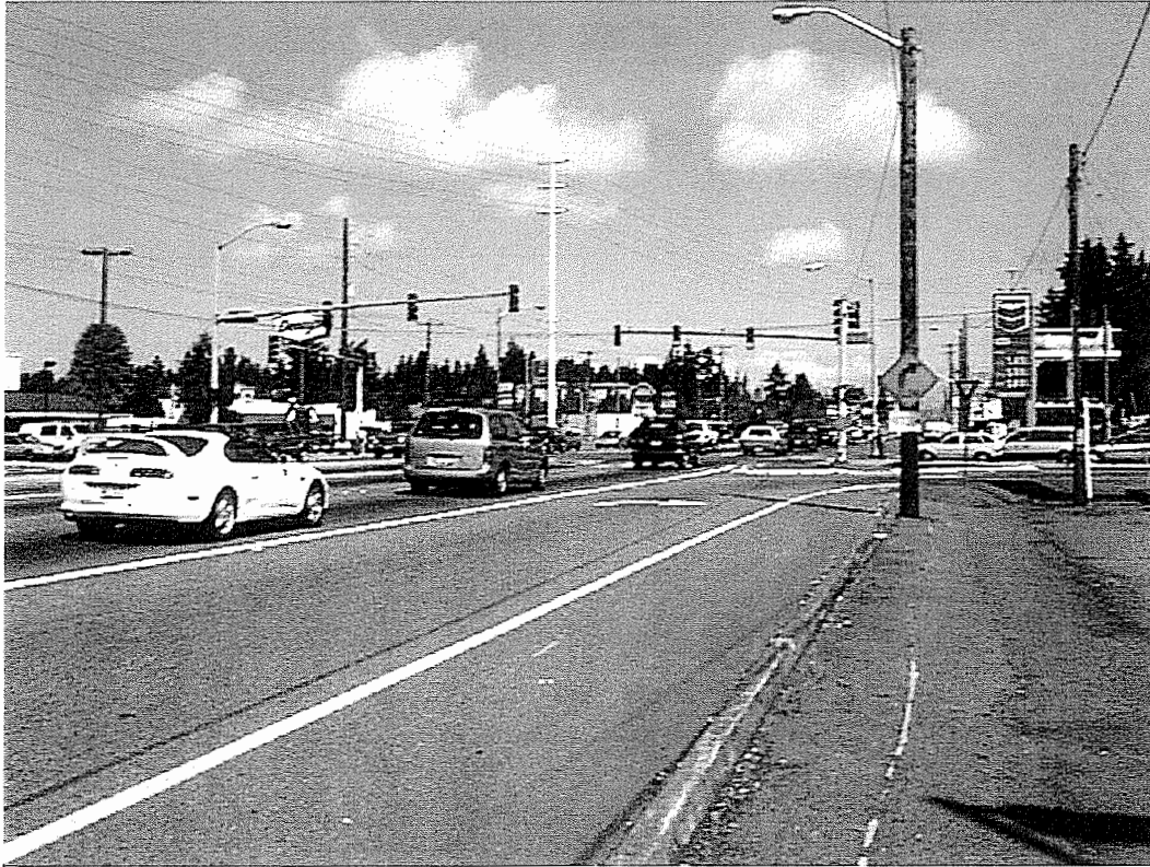
The pedestrian view looking north at the project's low point (North 155th Street) – a jumble of utility poles and street signage but no sidewalks.
