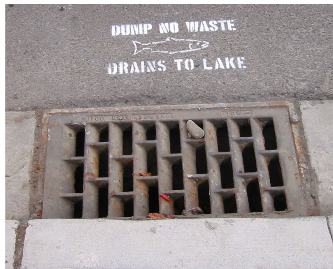
Storm Drain Maintenance Holes
