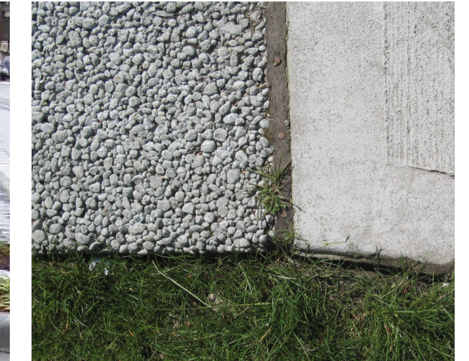
Porous Pavement (left)
