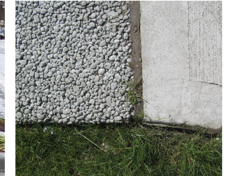
Porous Pavement (left)
