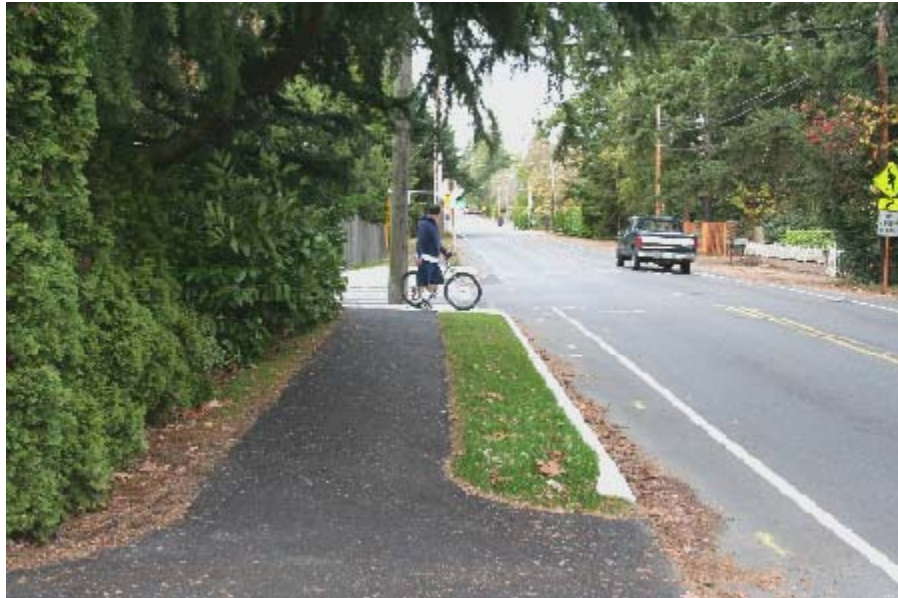
8th Avenue NW looking north at NW 190th Street
