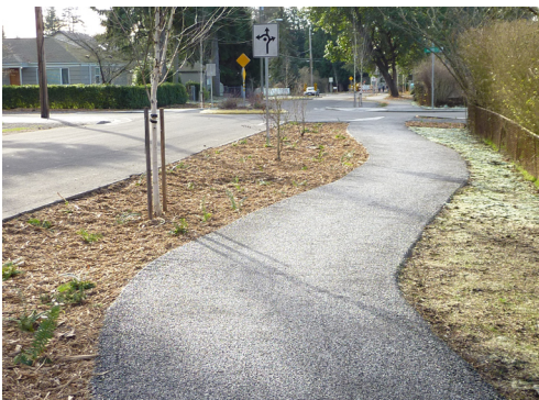
17th Ave NE between 145th and 150th Streets bioretention cells, porous pavement
