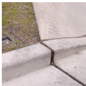
soil compaction near driveway
