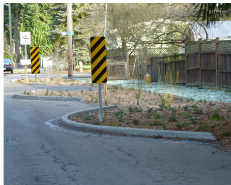
17th Ave NE between 145th and 150th Streets bioretention cells, porous pavement
